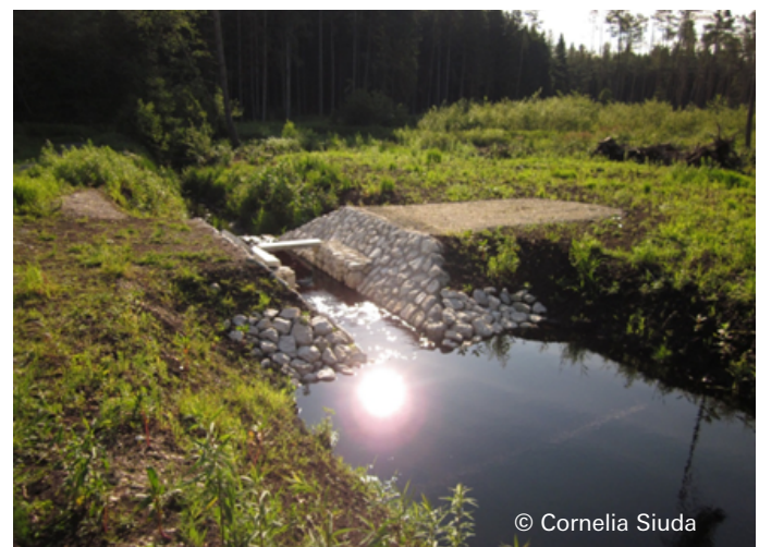
Mineral dam after completion
