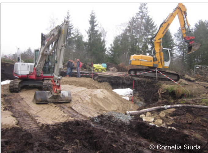
Compression of mineral material; right: Hose for water management
