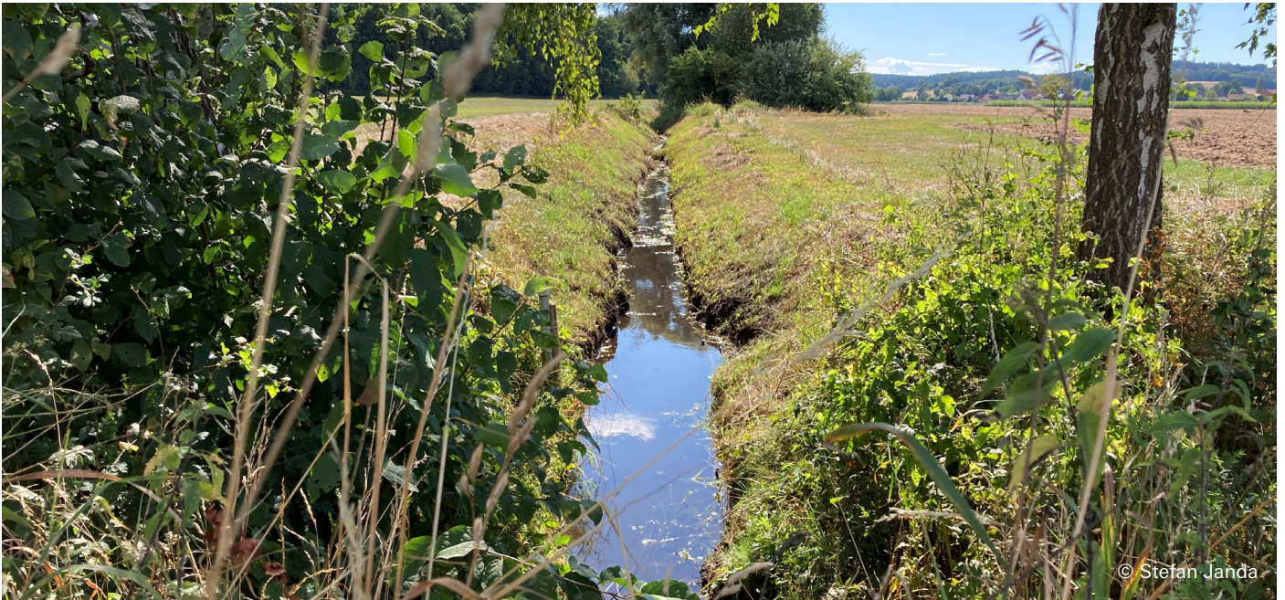
The Scheidegraben in the Schorner Röste - a typical drainage ditch in the Donaumoos.
